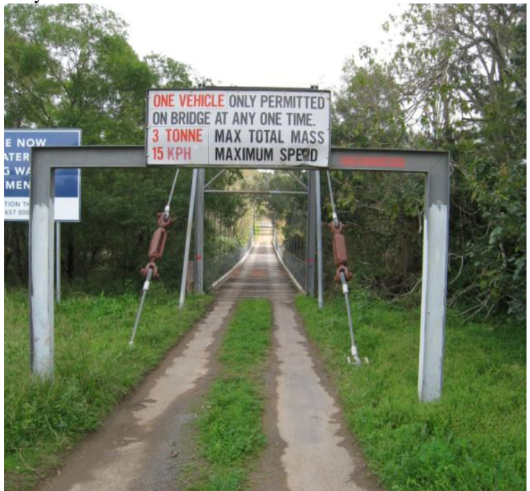
The suspension bridge
