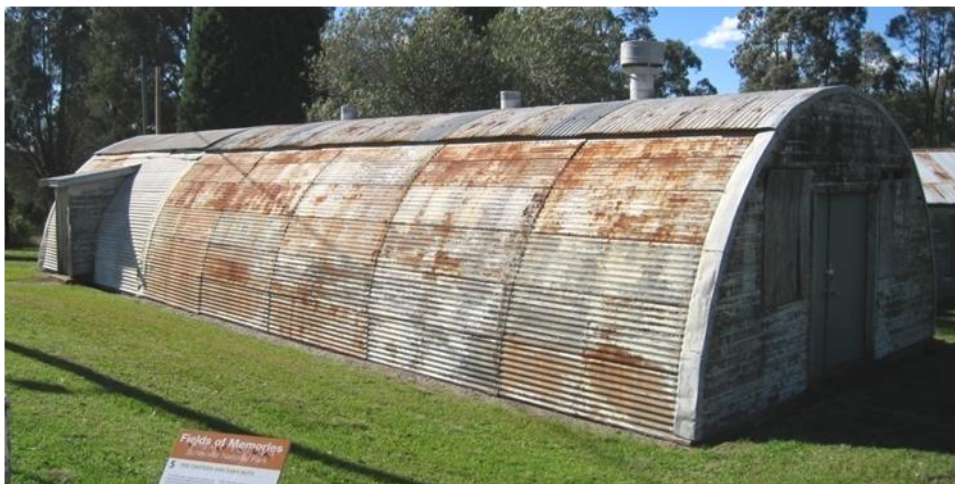
A Quonset hut, an American hut inspired by the British Nissen hut. Known as an SSAR hut, because it is built with Stran-Steel Arched Ribs.
