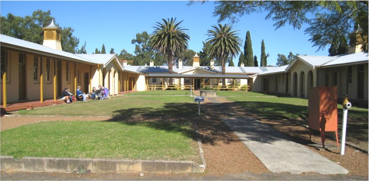
This complex was built in 1929 as new accommodation for the Dreadnought Farm. The far building was the kitchen and dining hall. The buildings on either side of the courtyard were used as dormitories. The buildings have been restored externally but still to be restored internally.
