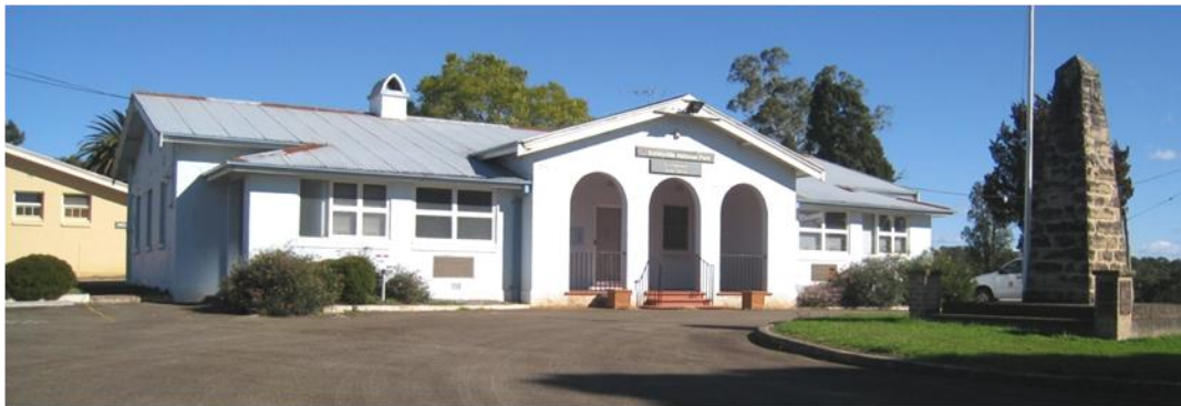
This building is now used by the Hills Sub District Office of the National Parks and Wildlife Service.
