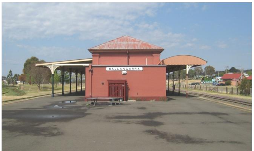
Wallangarra Railway Station. As it is on the border of NSW & Qld the left hand awning is NSW design & 4' 8½" gauge, while the right hand awning is Qld design & 3' 6" gauge.
