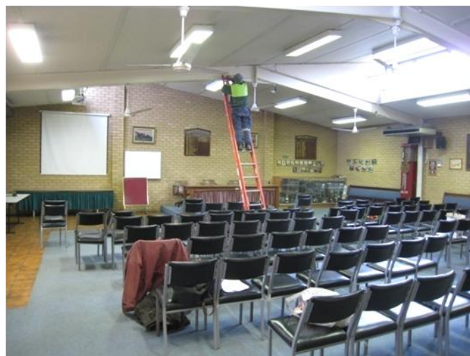
Neil cleaning the steel beams
